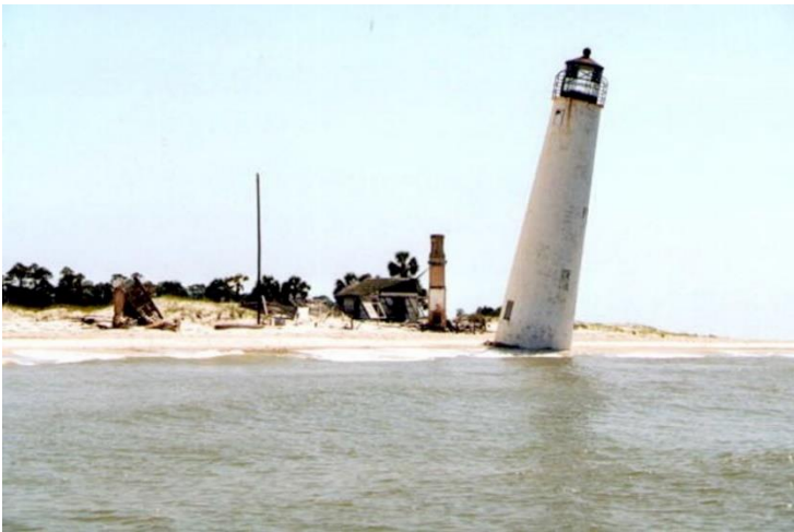
Mid-19 th century Cape St. George Light in 1999 before it collapsed in 2005 due to storm surge worsened by sea level rise. St. George Island. Image in public domain.
