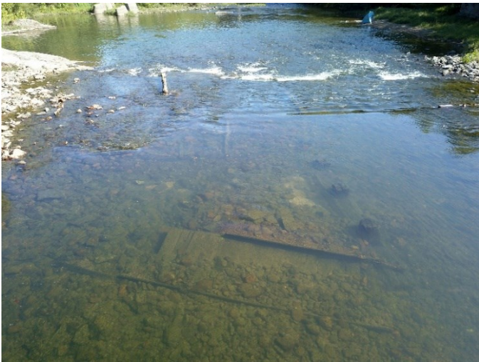
This small ferry came from the uppermost reaches of the Maury River in Rockbridge County. Likely washed from its moorings by a flood, it was dashed against these 19 th -century bridge pilings and was exposed after the removal of the Jordan's Point Dam. It is a rare example of a Shenandoah Valley small ferry and retains its iron rings used to fasten it to an overhead cable.
