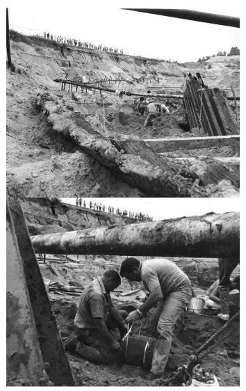
Bertrand excavation in progress. Large pipes are part of the system of well points used to keep the excavation dry. Original photo credit: United States Department of the Interior. Cecil W. Stoughton, 1969.
