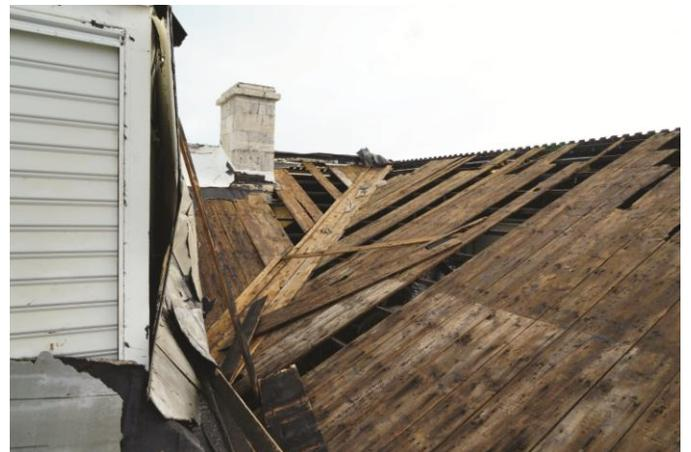
*Exposed wooden roof cladding.*
