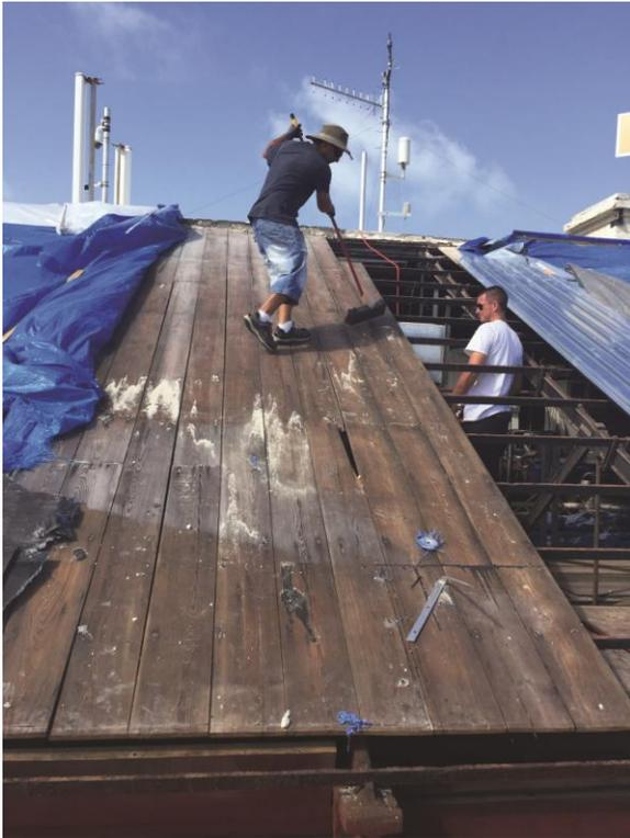
*Stripping wooden roof planking.*
